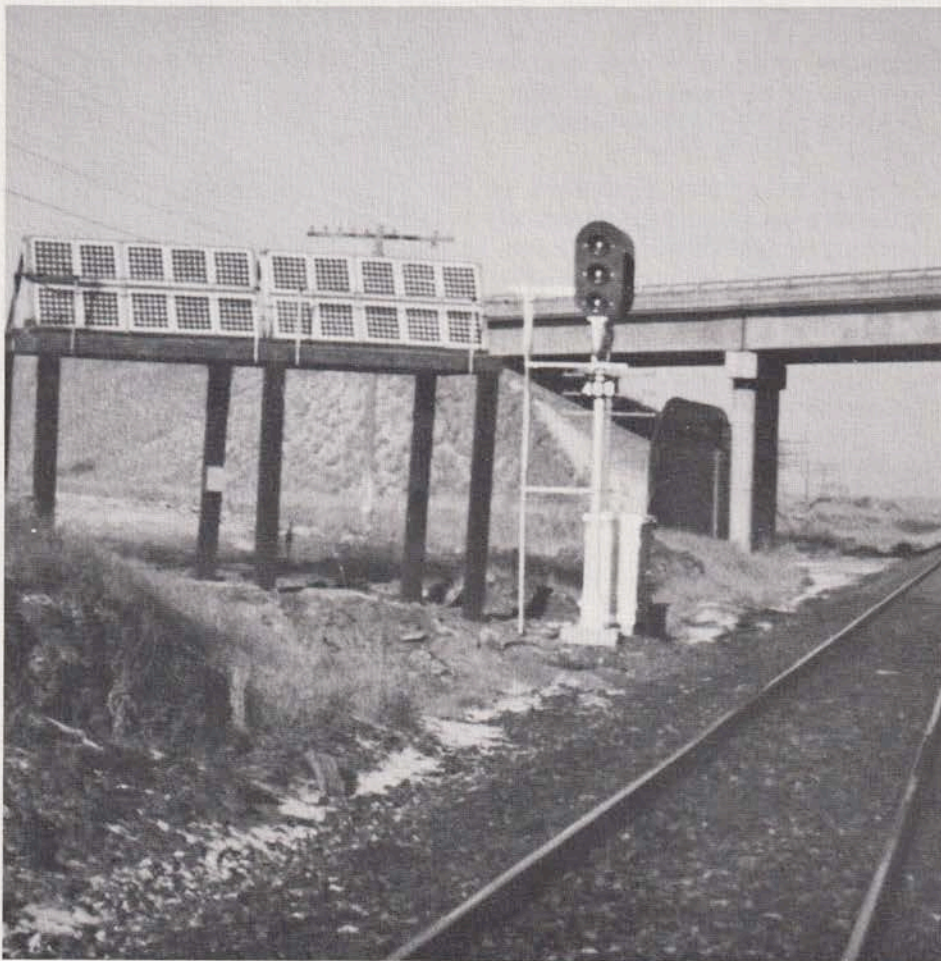
A 400 watt Solarex photovoltaic array provides power for track code units and intermediate signals near Spokane, Washington.
