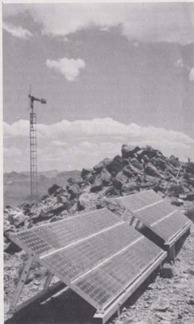
(Above) Basic 10W (peak) output solar panel comprised of 3" diameter Chevron™ silicon solar cells. This Solarex panel is a basic building block for large arrays. (Right) 460W (peak) solar electric system powering microwave and VHF repeaters in the Mojave Desert.
